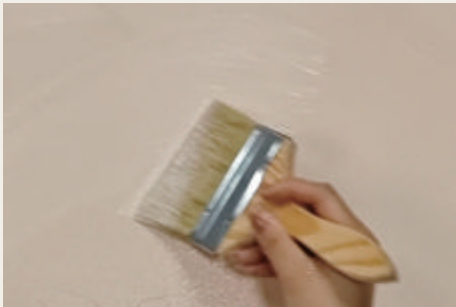
④ Brush the walls 1-2 times with a non-standard method.
