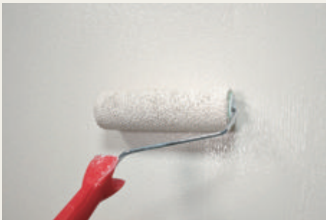
② Evenly apply the sealing primer, and the bottom layer should be completely waterproof after brushing.
